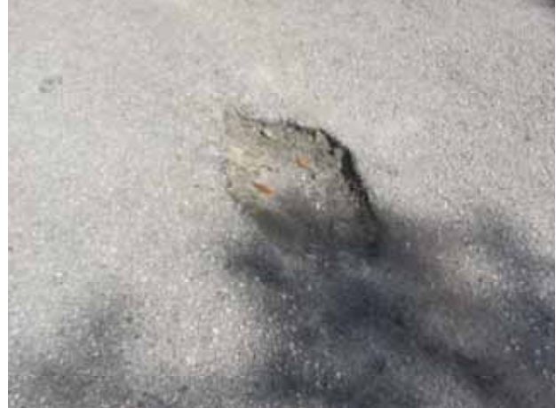
Asphalt pavement at clubhouse – Note pothole Asphalt pavement at clubhouse – Note pothole
