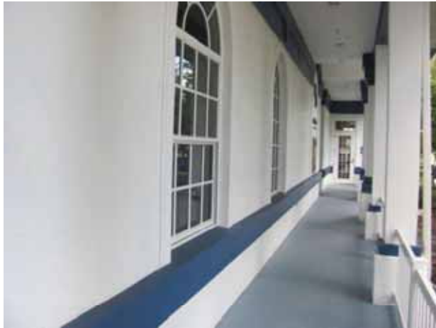
Painted stucco at clubhouse
