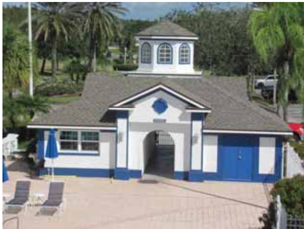
Pool cabana building
