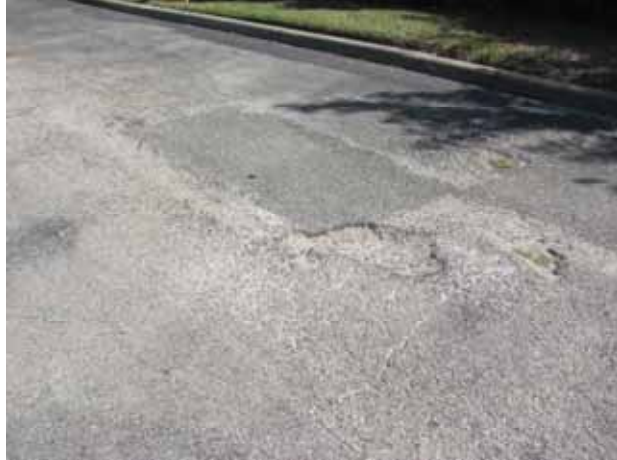
Asphalt pavement at clubhouse – Note pothole Asphalt pavement at clubhouse – Note pothole
