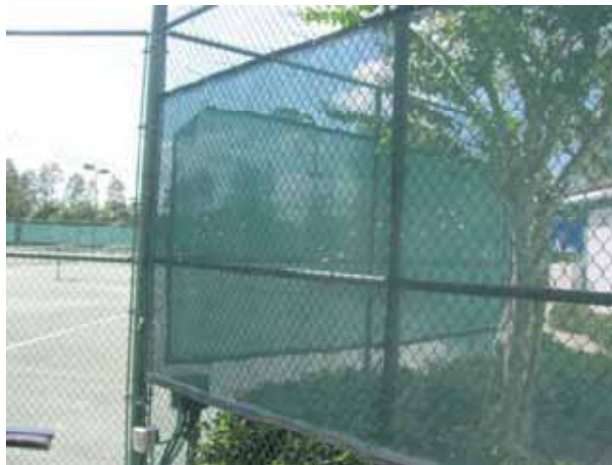
Tennis court fence
